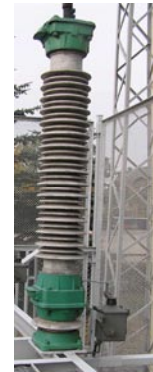
Fig. 4. GXA106 surge arrester with hydrophobic coating
