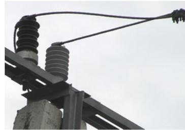
Fig. 2: Polymer concrete insulator (on the right) and porcelain insulator of 20 kV line.
