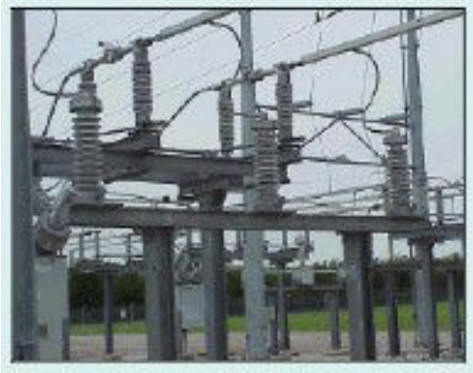
Figure 5. Intermediate station class arrester
